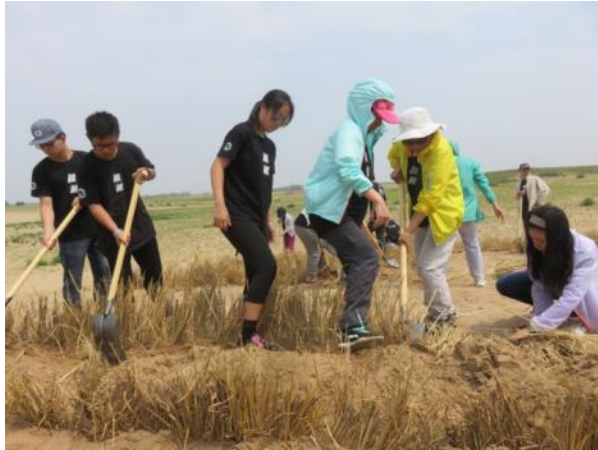
Paving straw-checkerboard
