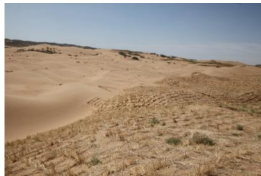
After paving straw-checkerboard
