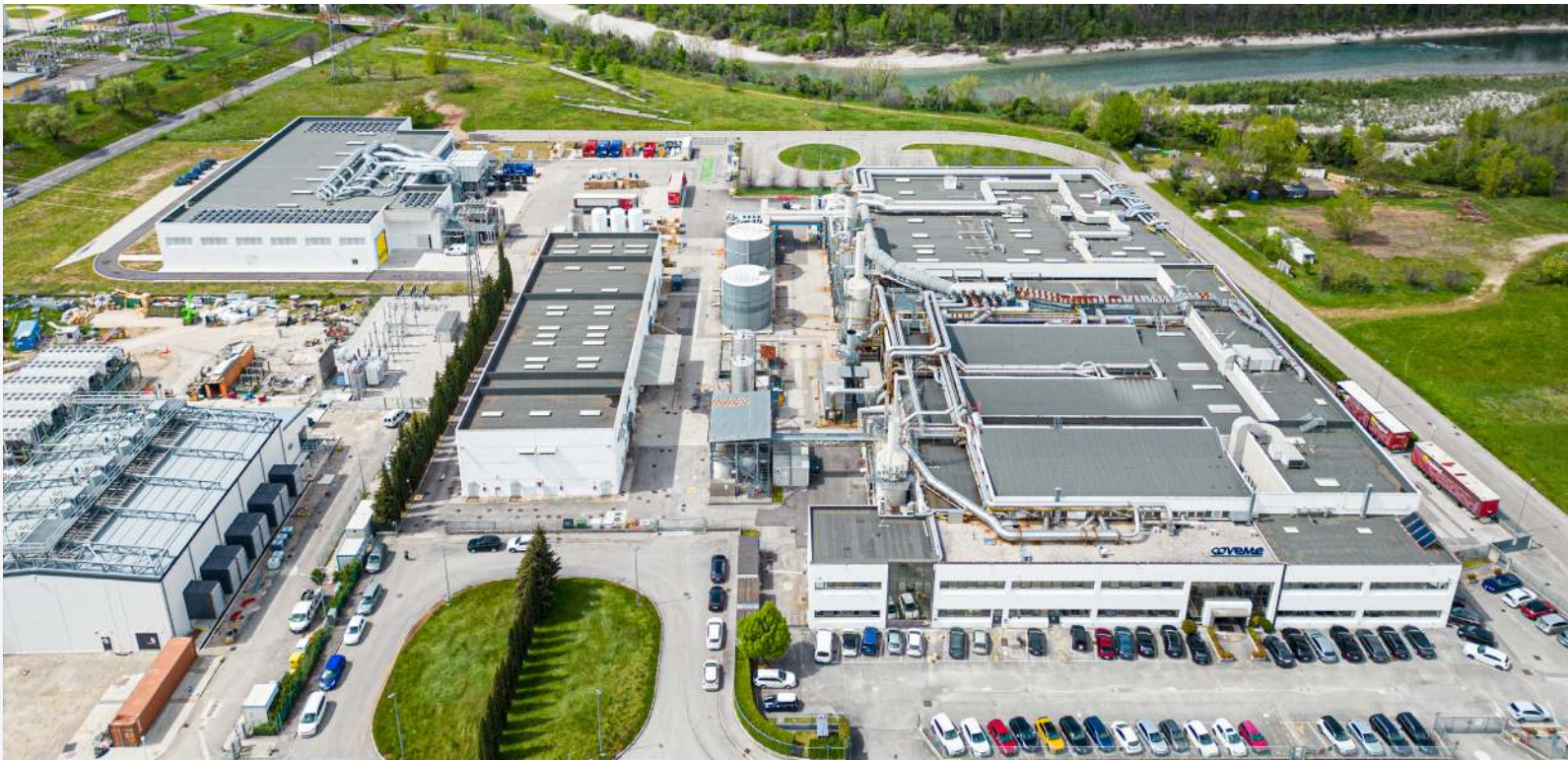
Coveme production plant in Gorizia
